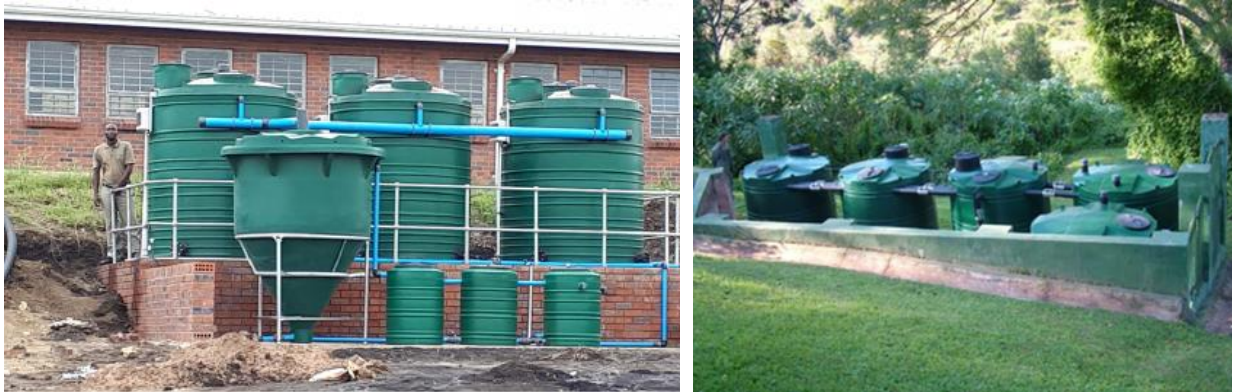
Figure 1: Examples of STP plants that have been used in other facilities ( Inchinga Hotel and Mona Primary school) in South Africa
