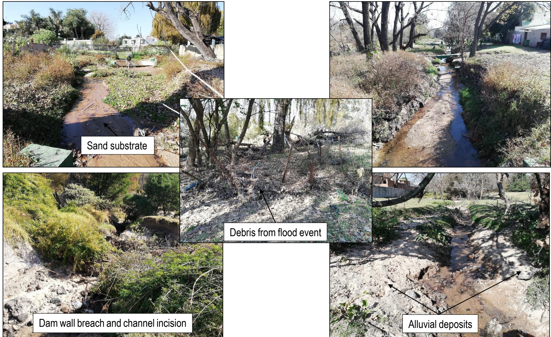
Figure 17: Illustration of the current condition of the Rip01 riverine system.
