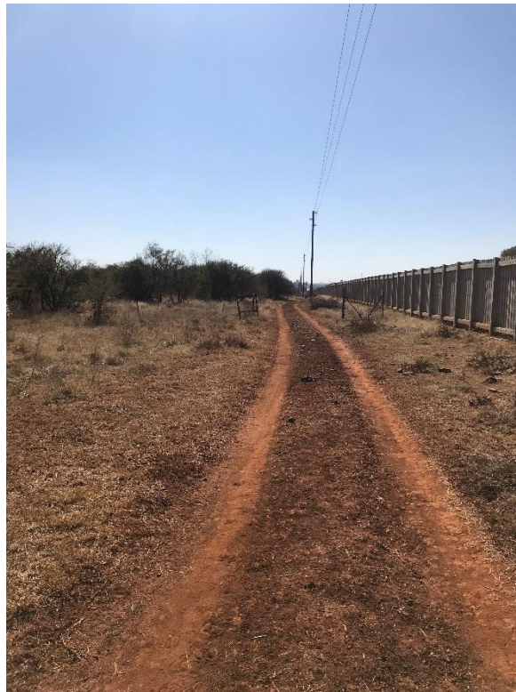
Figure 32: Access Road and Eastern boundary fence
