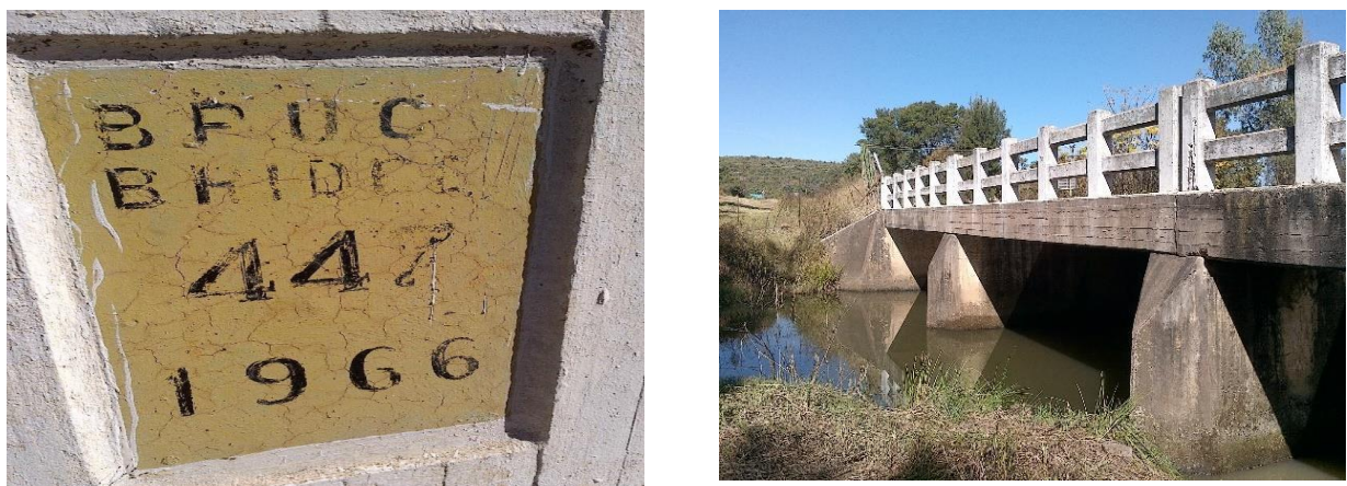
Figure 30: Groot Nyl River Bridge (HCAC, 2021)
