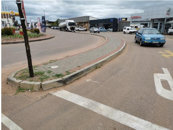
Figure 8: Pedestrian walkway at the start of the project
