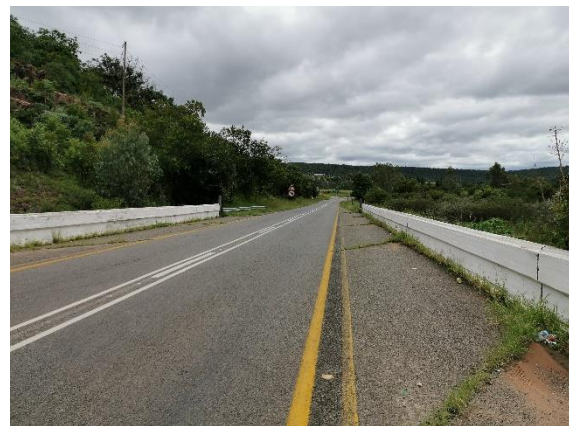
Figure 11: Existing bridges to be replaced
