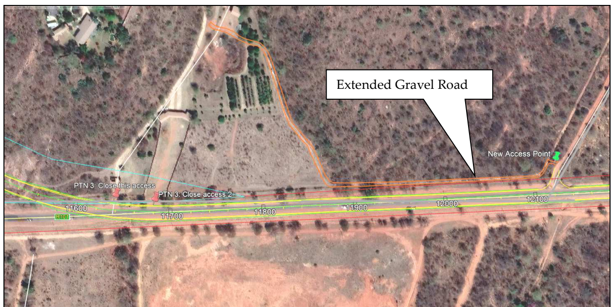
Figure 4.7: REM of PTN 3 new access and gravel road
