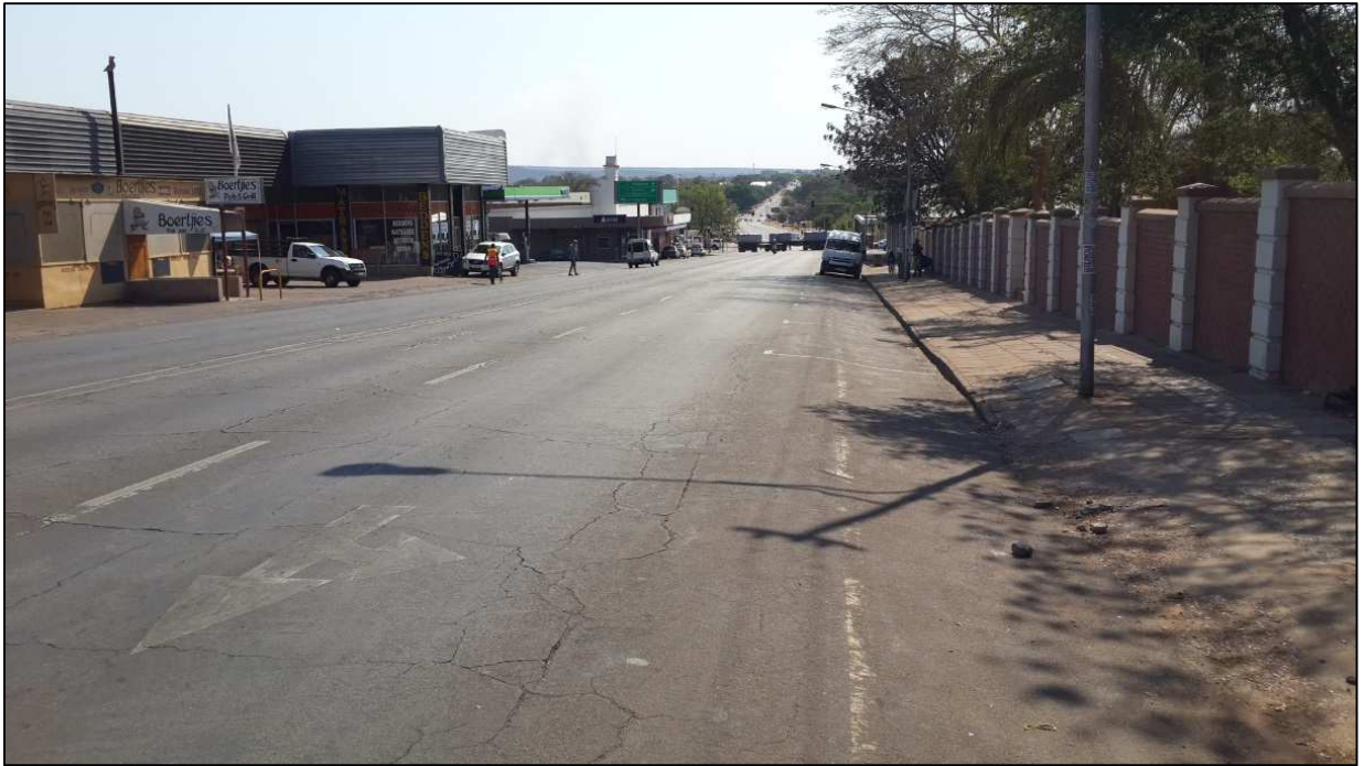
Photo 7.11: Parking bays on the right hand side km 26.60 to km 26.75
