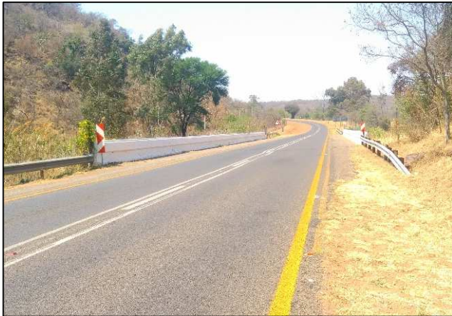
Figure 11.2: Approach to Bridge B375
