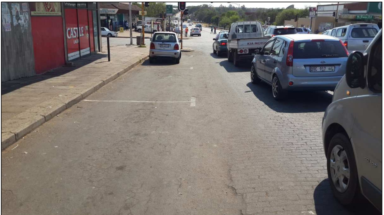
Photo 7.12: Concrete block pavers at km 26.80
