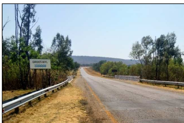
Figure 11.4: West approach to Bridge B447
