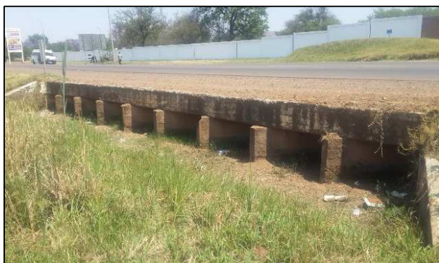
Figure 11.6: View of outlet
