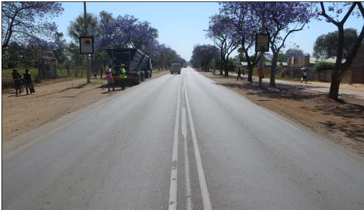
Photo 7.1: Typical appearance of first section at km 0.20
