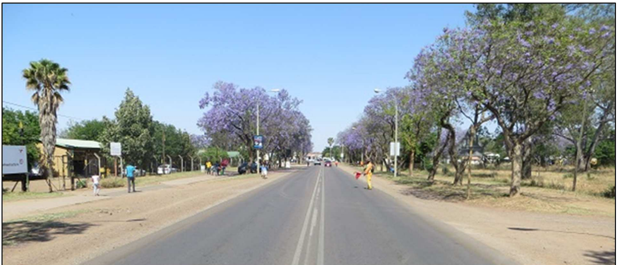
Photo 13.1: Street light fittings in opposite arrangement in Bela Bela
