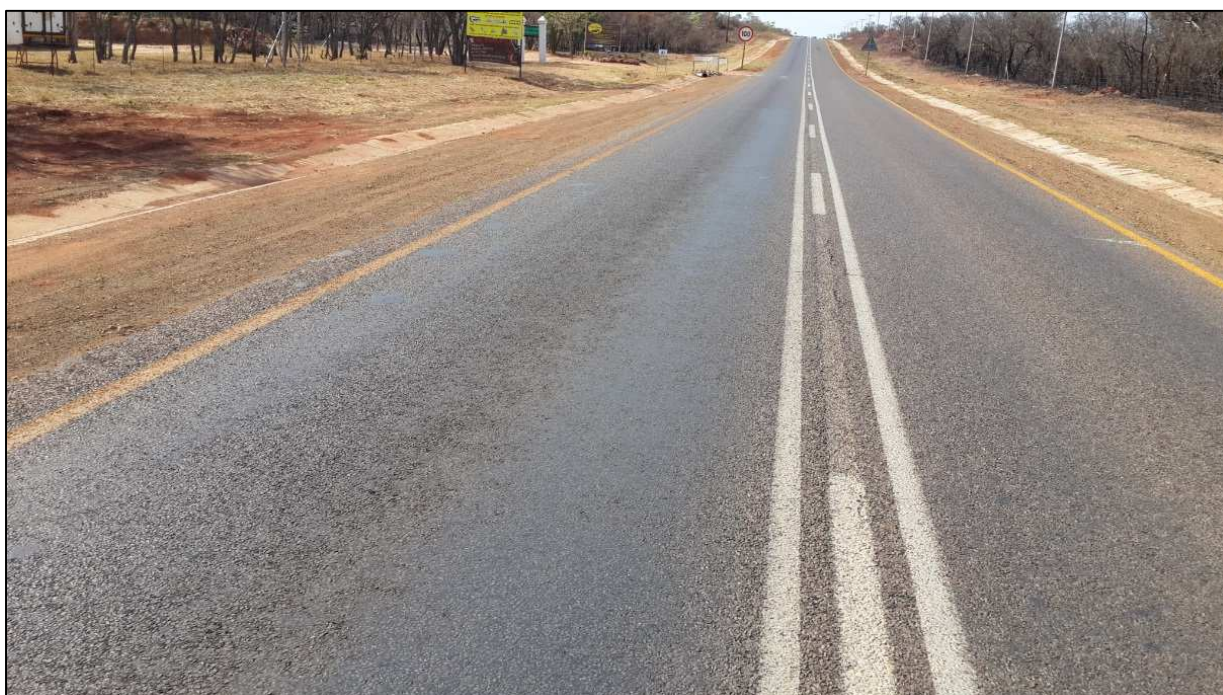
Photo 7.6: General appearance of section from km 5.44 to km 25.05 with flushing
