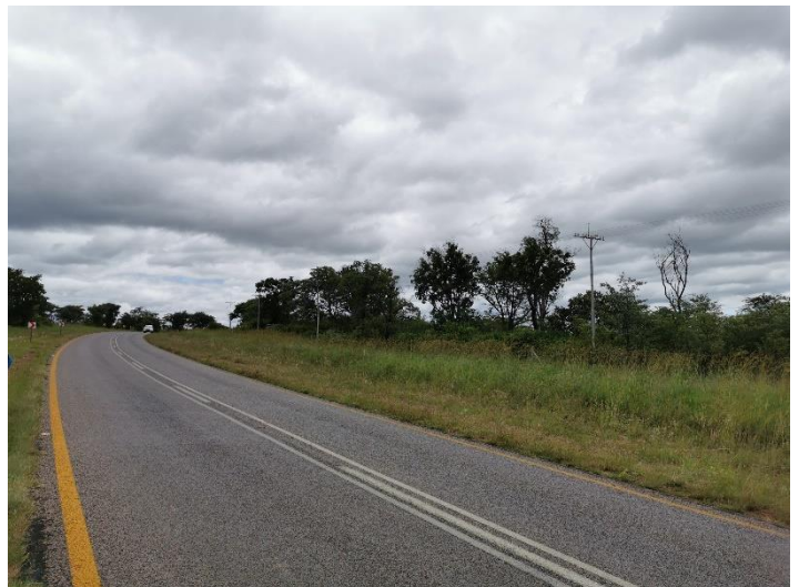
Realignment Area 3 also with a fair to good pavement condition
