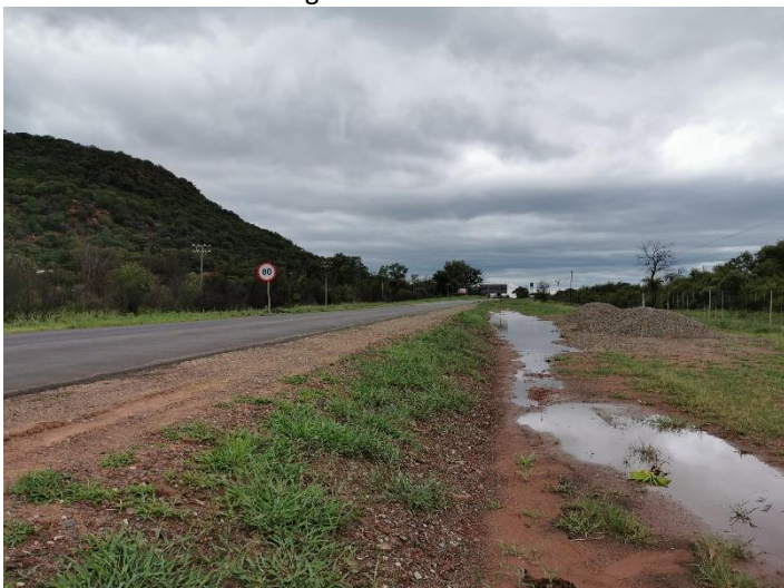
Exiting road servitude consists mainly of gravel shoulders bounded by fences on both sides
