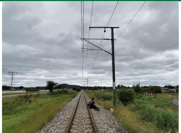
Transnet railway line parallel to the road in Bela Bela
