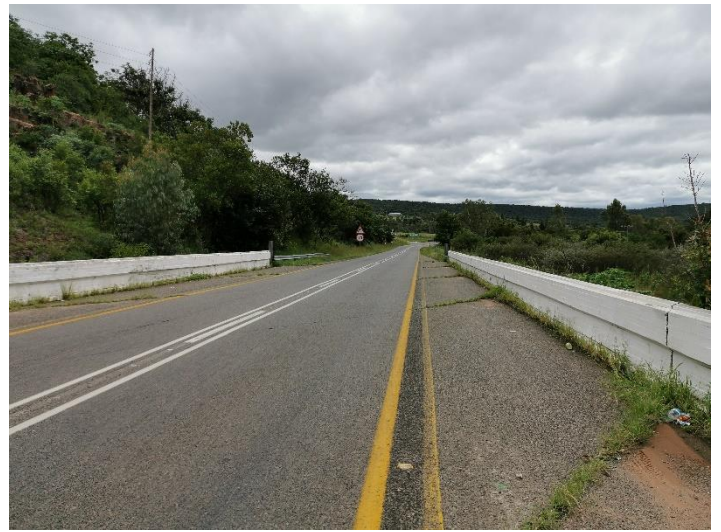
Modderloop Bridge with ageing infrastructure
