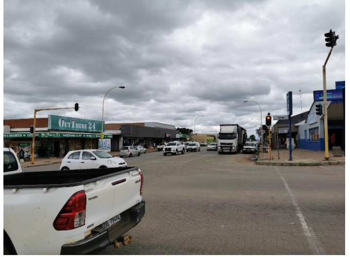
End of the project in Modimolle at the intersection of the R101 and R33 (km 26.8)
