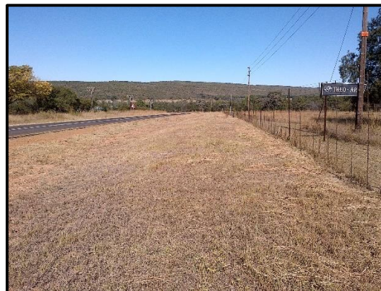
Figure 7.8: Conditions along the road widening sections.
