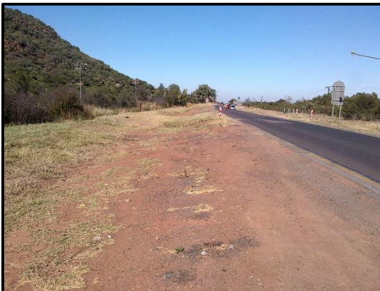
Figure 7.9: Conditions along the road widening sections.
