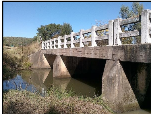
Figure 8.16: Eastern elevation of Bridge 447.
