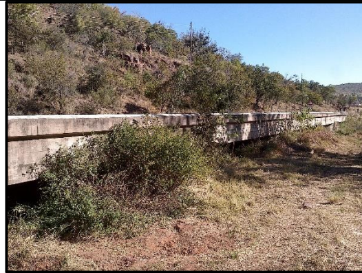
Figure 8.14: Eastern elevation of Bridge 375.
