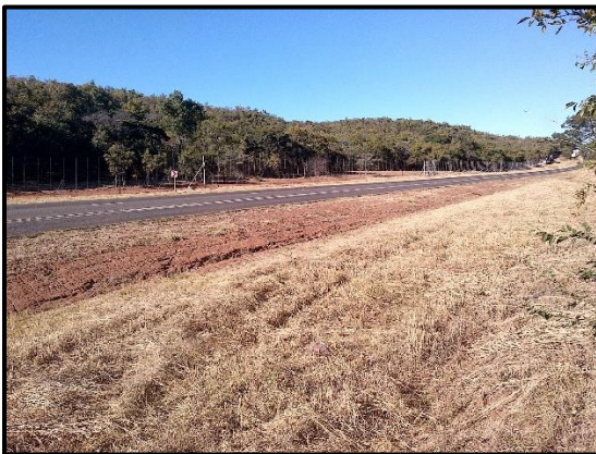
Figure 7.7: Conditions along the road widening sections.
