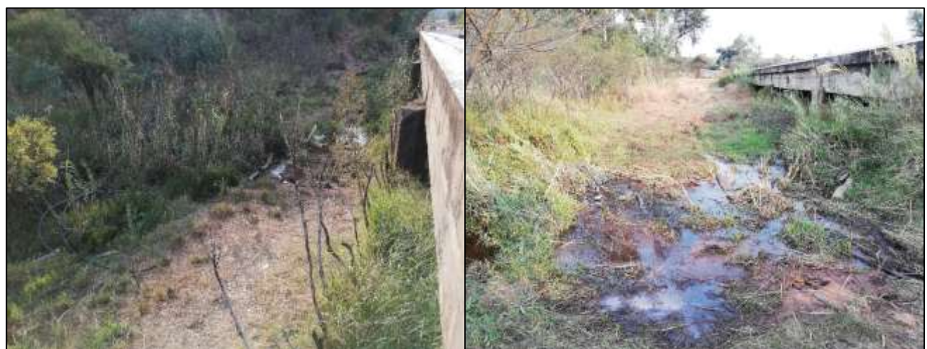
Figure A04. Representative images of CVB02 at the existing R101 crossing.
