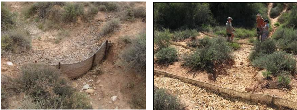
Figure 6: Example of erosion control fences
