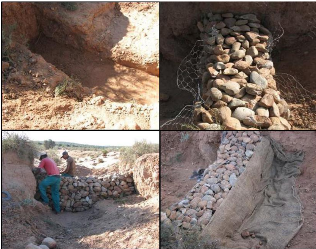
Figure 8 Trench digging and lined with wire netting and gabion stones
