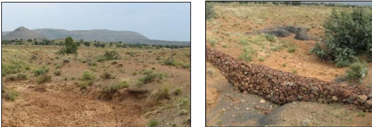
Figure 7 Site highlighting severe gully erosion due to increased stormwater runoff and rehabilitation after the installation of a functional stone gabion
